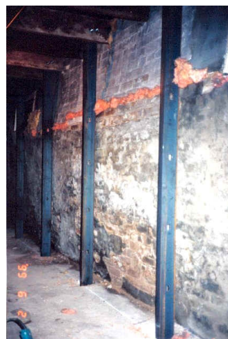
Some examples of bracing using steel members
