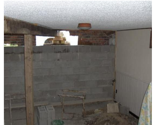
One basement wall undergoing complete replacement
